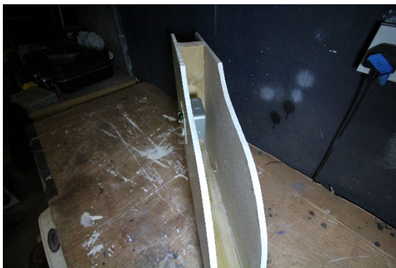
Figure 3 - MyHome socket inside wall partition
